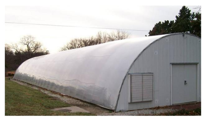
Figure 1. Double poly Quonset-style greenhouse with solid north end wall.
