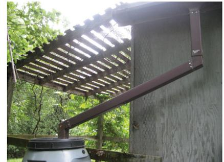
Figure 2. Downspout extension directs rainwater into the rain barrel.
