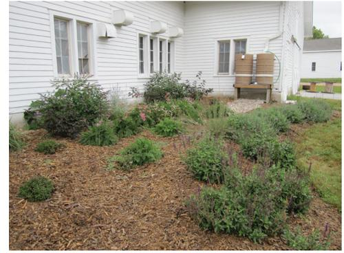
**Figure 7.** Overflow water directed to a rain garden. Gravel below overflow reduces soil erosion.
