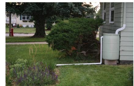
Figure 5. PVC extension connected to overflow to direct water away from barrel.
