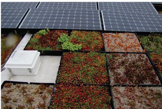
Figure 6. Green roof planting methods include trays (left) and seeding/plugs (right).
