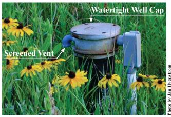
Figure 3. A watertight, secure cover caps the top of the well.
